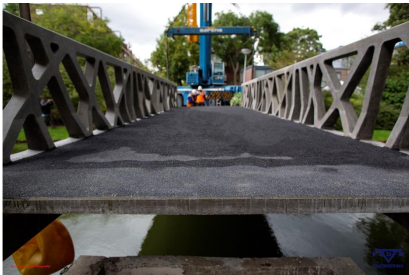
Figure 4: Deck thickness of bridge only 60mm
