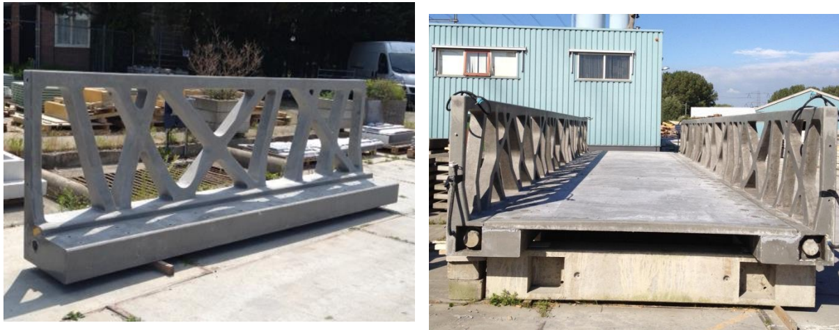
Figure 5: The 4.3m long handrail element (left), and post-tensioned elements (right)
