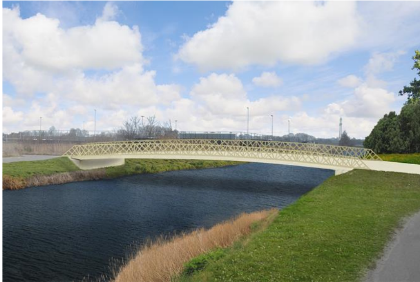
Figure 13: Current design of the Ultrabridge in Eindhoven, The Netherlands, with the highest concrete strength in the world. The compression cubic strength of concrete will be up to 300N/mm 2 .
