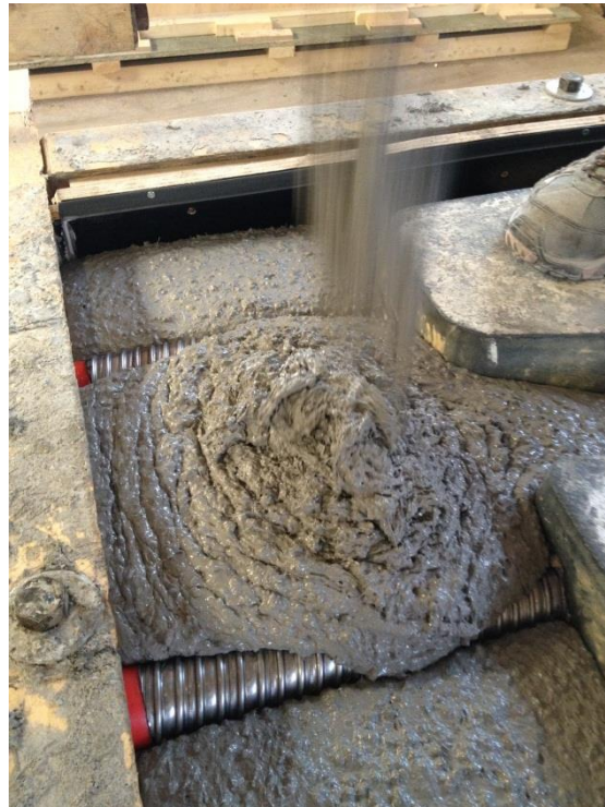
Figure 6: Low w/c ratio makes the concrete thixotropic
